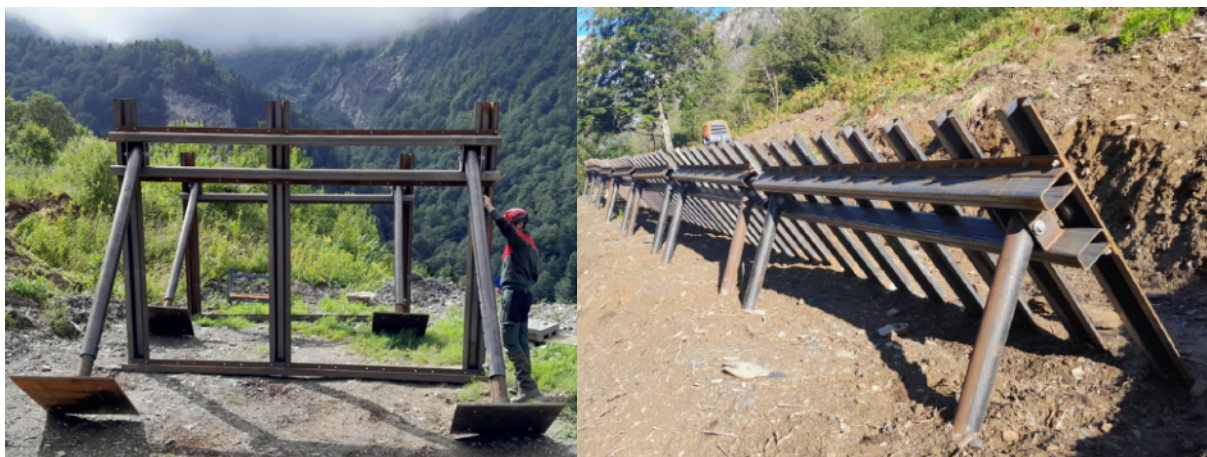
Figure 5 Snow bridge for Heli lifting (the crossbeams were removed to reduce weight) and view of the finalised structure.
