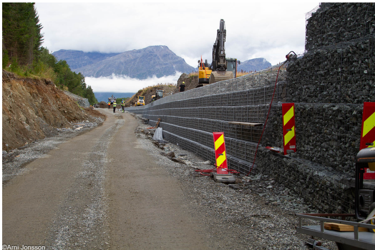
Fig. 5 The figure shows the 12 m high dam under construction. To the right is the 5 m high gabion wall. Photo taken in August 2023.
