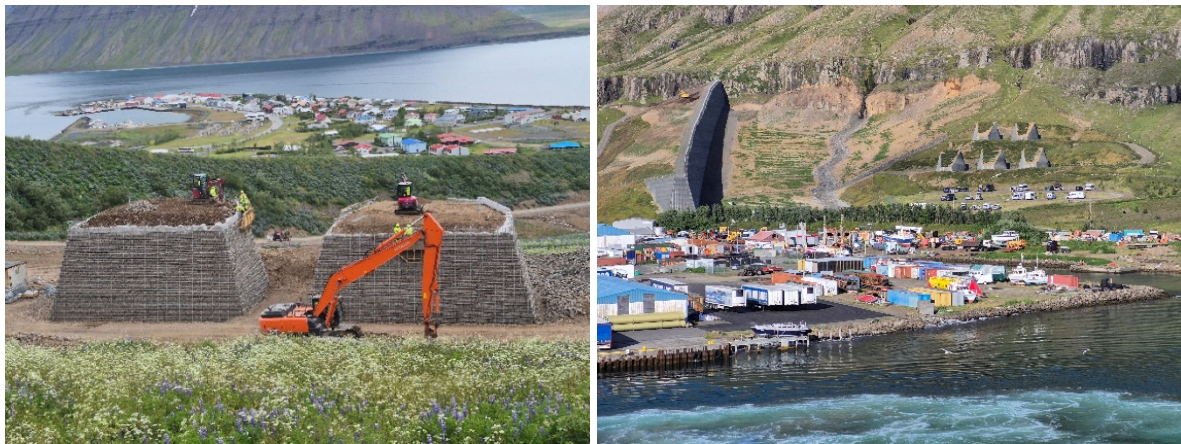
Figure 6 Left: The construction of two steep, 10 m high braking mounds upstream of the Flateyri, Innra-Bæjargil deflecting dam. Right: The recently finished, 9 m high braking mounds and the 18 m high deflecting dam below Kálfabotnar in Seyðisfjörður. Photos: Kristín Martha Hákonardóttir, July and August 2025.
