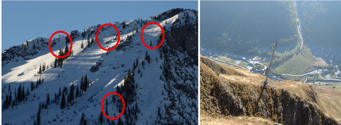
Figure 2 Left: Alta ski resort (USA) – towers are placed close together to directly affect individual release areas to mitigate hazard of (natural or human triggered) small avalanches which could reach ski slopes. Right: Samnaun (Switzerland) – 87 RACS are used to protect the access road, the settlement and ski slopes.
