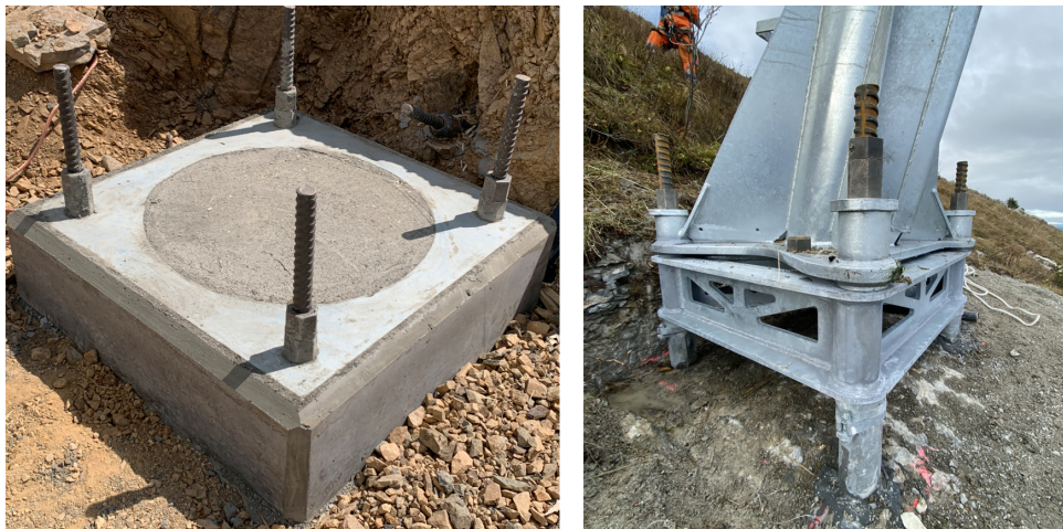
Figure 1 Wyssen concrete (left) and concrete-less foundation (right) with 4 vertical and 1 shear relief anchor.
