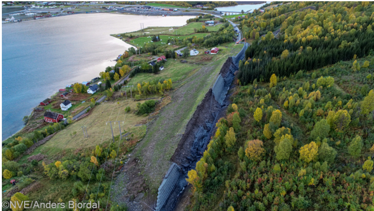
Fig. 1 This figure shows the catching dam at Samuelsberg Troms county northern Norway and the two locations of failure of the 12 m high facing side. Photo Anders Bjordal/NVE.
