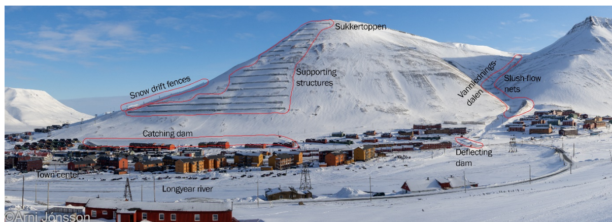
Fig. 2 Red areas in the figure show areas with constructions to mitigate the avalanche danger from Sukkertoppen and slush-flow danger from Vannledningsdalen. Photo taken on April 1, 2025.
