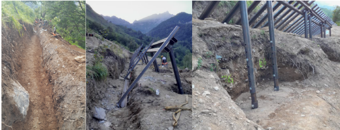
Figure 4 View of the earthworks for the installation of the structures
