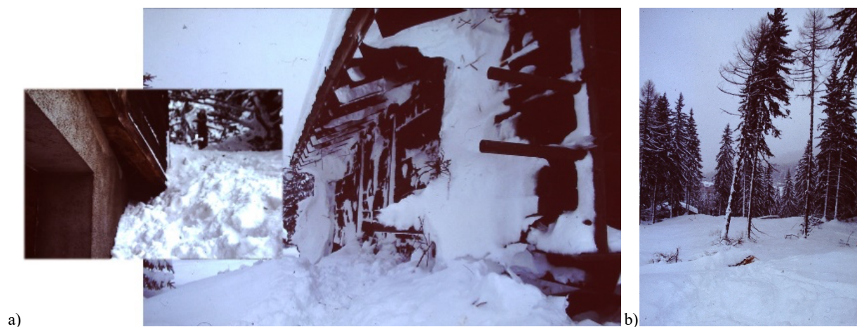
Figure 1.2 a) Example from La Fouly, Switzerland (1999), where the powder cloud exerted enough force to partially dislodge a wooden chalet from its foundation. b) "Flag trees" observed in the aftermath provide indirect evidence of the powder cloud's intensity and direction, offering insight into the avalanche's dynamics.
