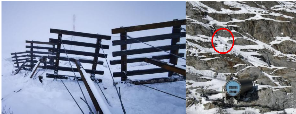
Figure 7 Left, view of the four modules located above the gondola bottom station (right)
