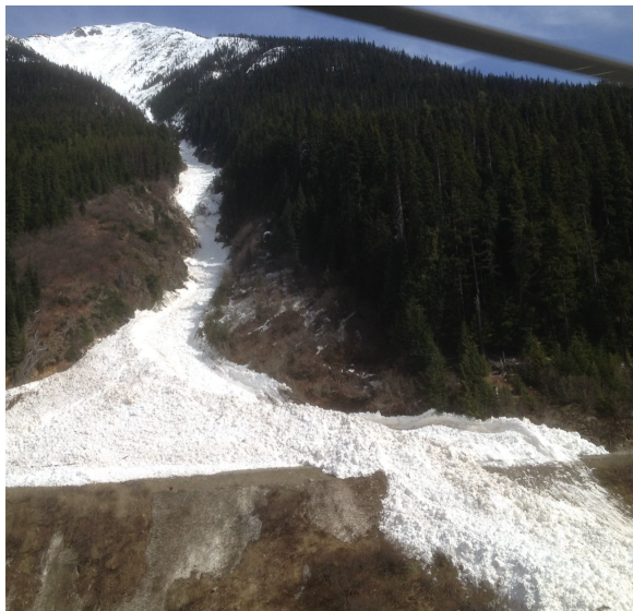
Figure 1 Explosive-triggered avalanche in Path 51, May 14, 2012 with debris accumulation visible along Highway 99 (Source: MoTT).
