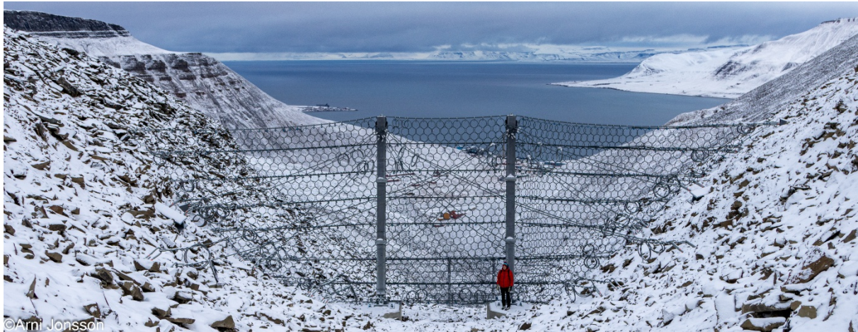
Fig. 4 This photo shows the valley's largest net, which stands 7 m tall on a 1 m foundation. The photo is taken on Oct. 2, 2024.
