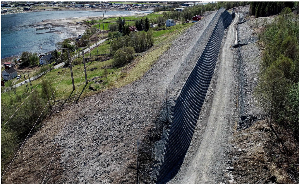
Fig. 6 The figure from July 2025 shows completed catching dam above the residential area in Samuelsberg. Photo: NVE/Anders Bjordal.
