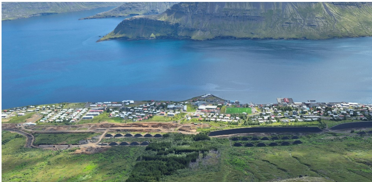
Figure 7 Protection measures above Neskaupstaður, East Iceland. From left to right: Construction site below Nesgil and Bakkagil. Ten 10 m high mounds below Nesgil have been constructed and foundation work laid for a 800 m long and 23 m high catching dam. To the right are 13 mounds below Drangagil, located upstream of the 17 m high catching dam. These protection measures were built in 1999 and interacted
