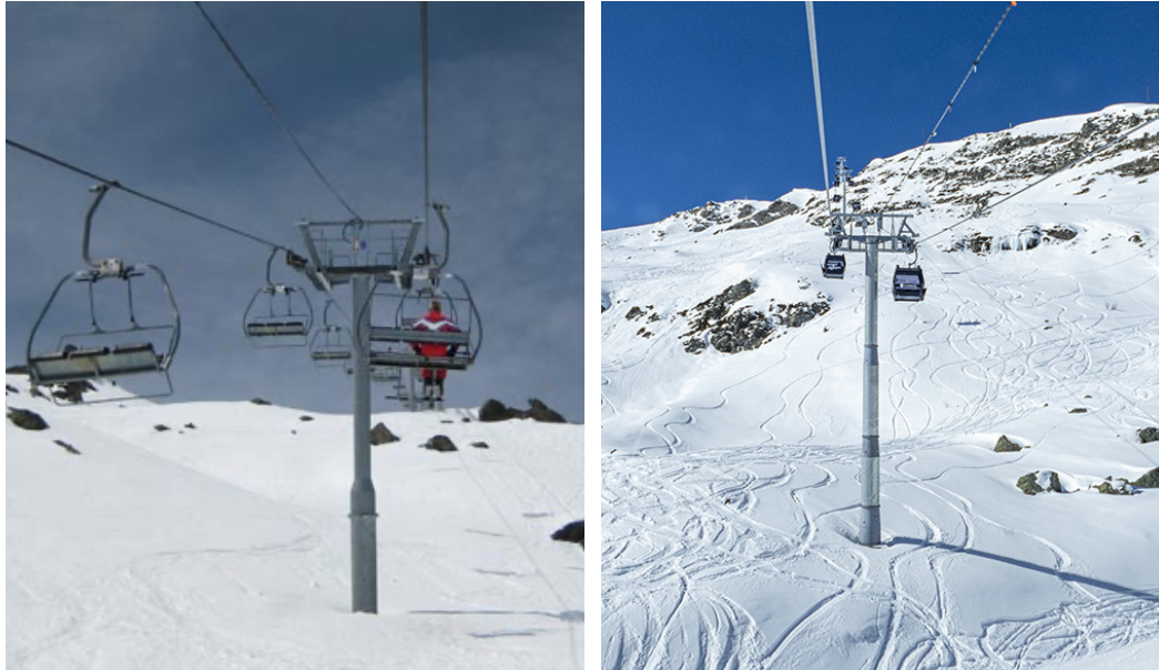
Figure 1 Left: typical design and size of a fixed-grip chairlift built in the 1980s (Creux Noirs at Courchevel). Right: modern gondola (La Masse at Les Ménuires)
